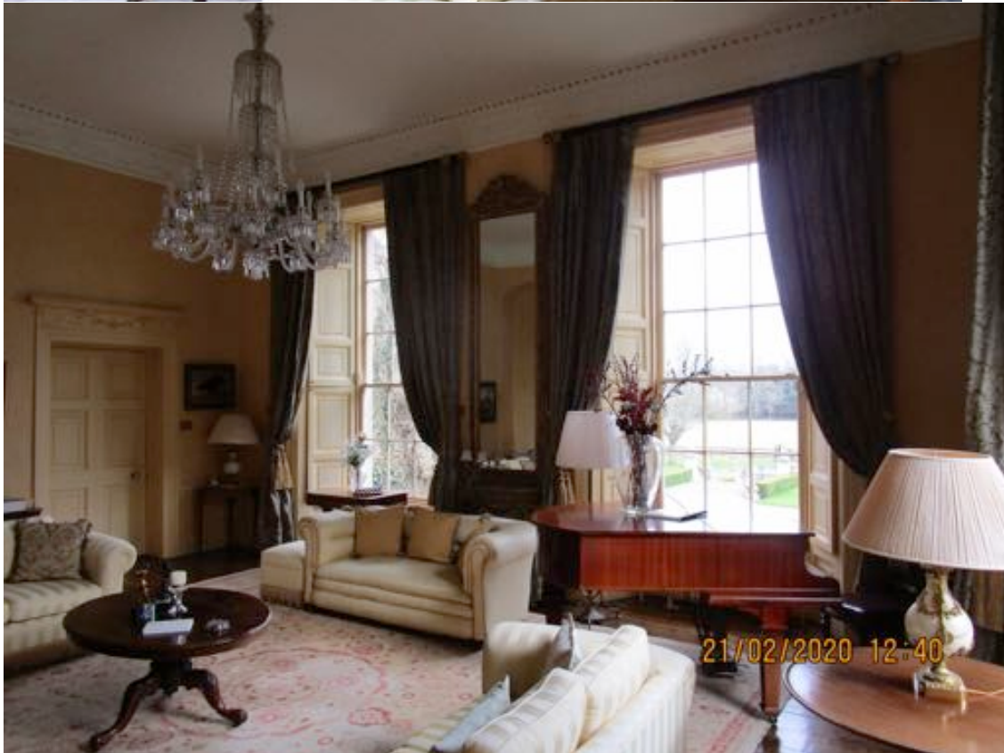
Fig 24 above and Fig 25 below) General view above of Drawing Room (GF-02) with excellent original joinery, plasterwork and chimneypiece.
