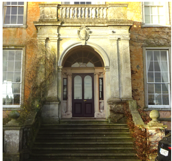
Detail above (Fig 6) of the dormer window with its prominent moulded pediment and unusual Wyatt type format and a detail of the open porch (above right Fig 7) and steps which were added most likely in the late 19th century or early 20th century.
