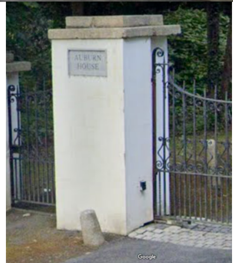
The entrance gates are in their original position with convex quadrant walls and are rendered masonry with plain granite cappings and modern wrought iron gates (Fig 80 – general view above and Figs 81 – detail of gate pier and Fig 82 – flanking wall)
