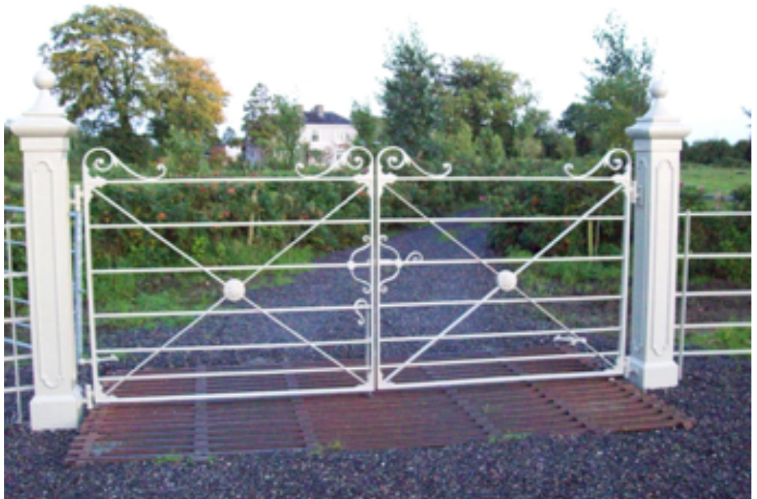
Fig 11 : Typology for the new entry gate to the fenced grounds attendant to Auburn House – this is consistent with the proposed estate fencing to be used (see Fig 10 above) and understated while marking the significance of the new entry point. Note: all fencing including new gates and gate piers to be painted black).
